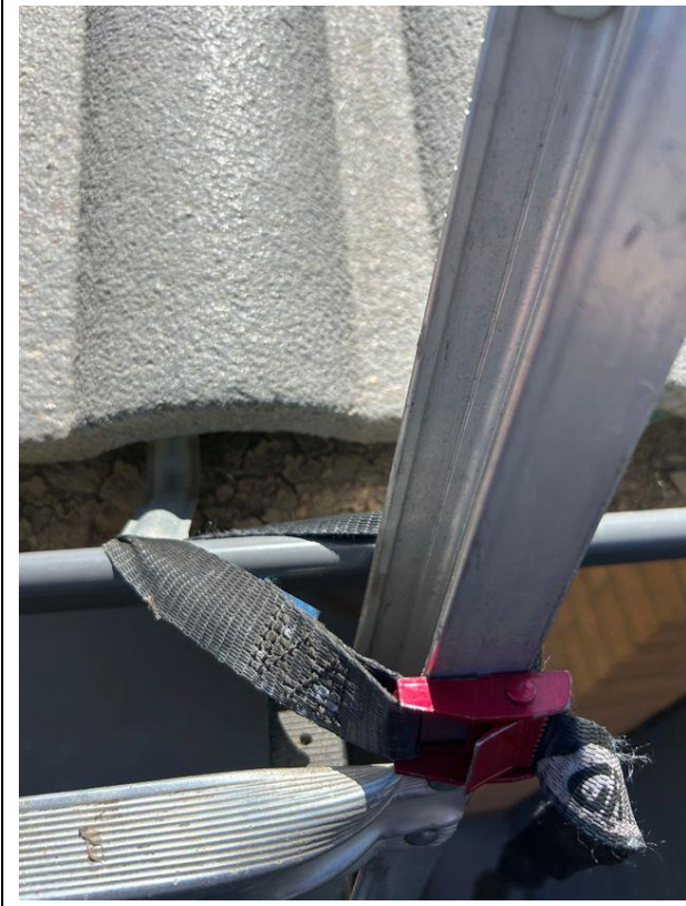
Ladder access safety tie off
